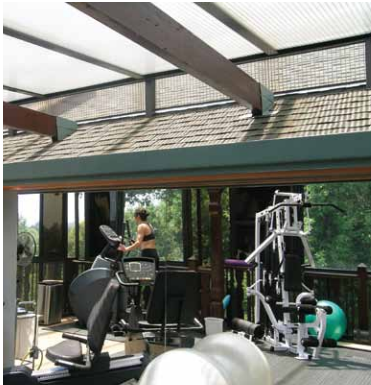
ABOVE LEFT: 3 mm ACRYLITE acrylic Wave Profile sheets create partitions while allowing an abundance of natural light at the Hamilton Health Centre in Hamilton, Ontario. ABOVE RIGHT: Personal training studio is covered with 16 mm ACRYLITE Double-Skinned sheets in the Monterey Peninsula. Design/Build: RBCO, California.
