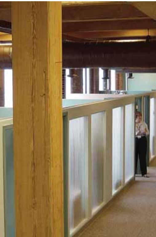
ABOVE LEFT: 3 mm ACRYLITE acrylic Wave Profile sheets create partitions while allowing an abundance of natural light at the Hamilton Health Centre in Hamilton, Ontario. ABOVE RIGHT: Personal training studio is covered with 16 mm ACRYLITE Double-Skinned sheets in the Monterey Peninsula. Design/Build: RBCO, California.
